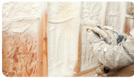
PU/PIR Spray Insulation with custom thickness and density
